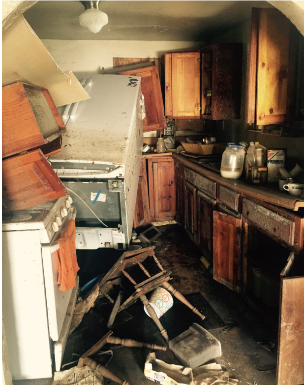
Photo of a flooded family home, the day before it was demolished. Presbyterian Disaster Assistance Mission Trip Beaumont, Texas. Photo by Jeanie Shaw
